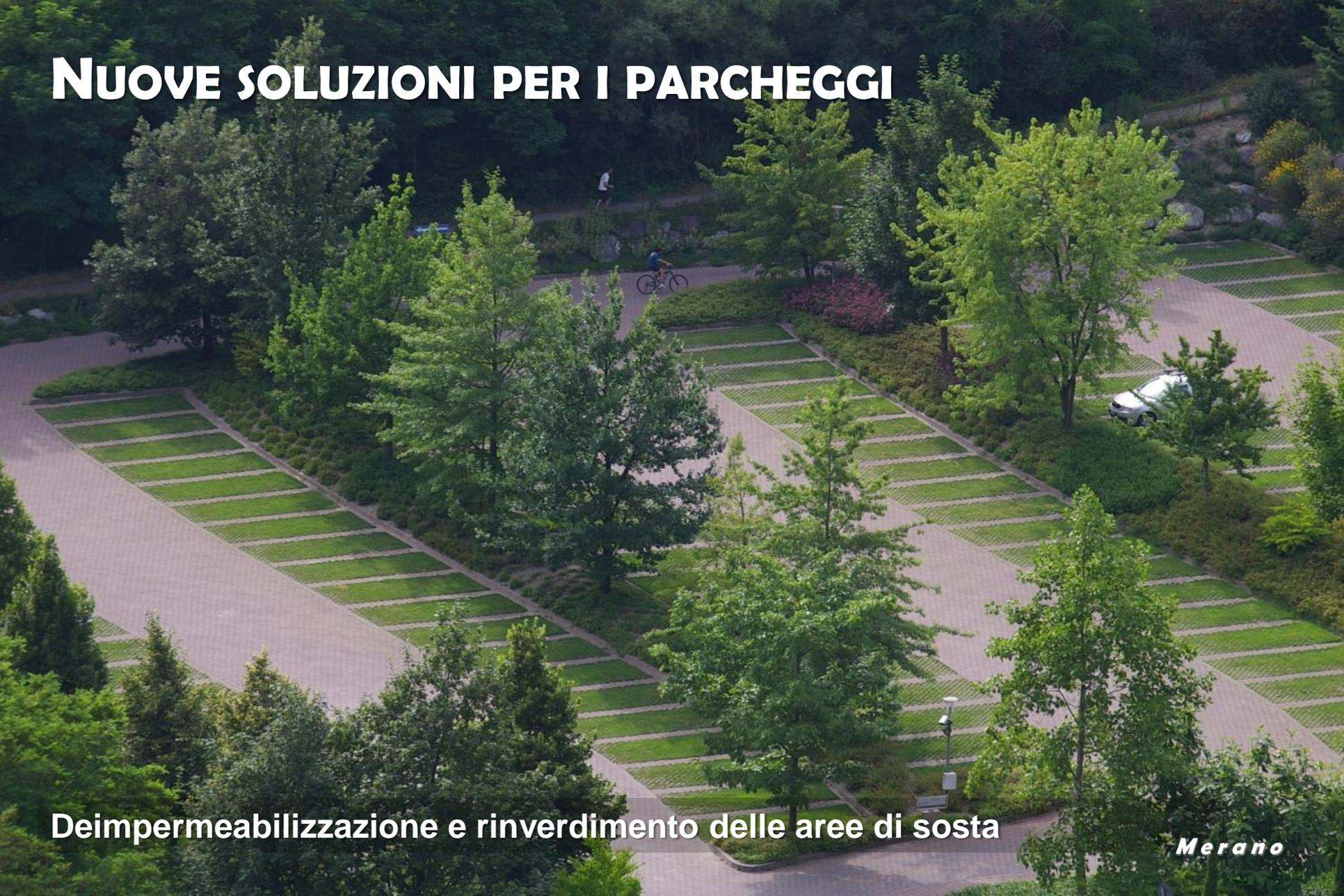
An aerial photograph of a parking lot designed with permeable paving and integrated greenery. The parking spaces are rectangular and filled with a light-colored, textured material, likely permeable concrete or pavers. Between the parking spaces, there are rows of young trees and low-lying plants. A paved path runs through the center of the lot, where a person is walking and another is riding a bicycle. A white car is parked on the right side. The background shows a dense forest of tall trees.
